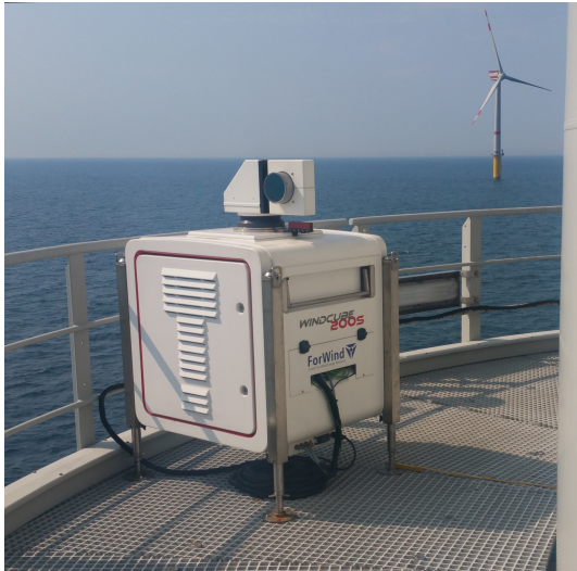
Figure 3. Lidar system Windcube 200S on the transition piece of wind turbine GT58 in the offshore wind farm Global Tech I. On the right side of the image the tower of the turbine is visible while turbine GT51 northwest of GT58 can be seen in the background (cf. GT I layout in Fig. 2) (Stephan Voß, ForWind).
